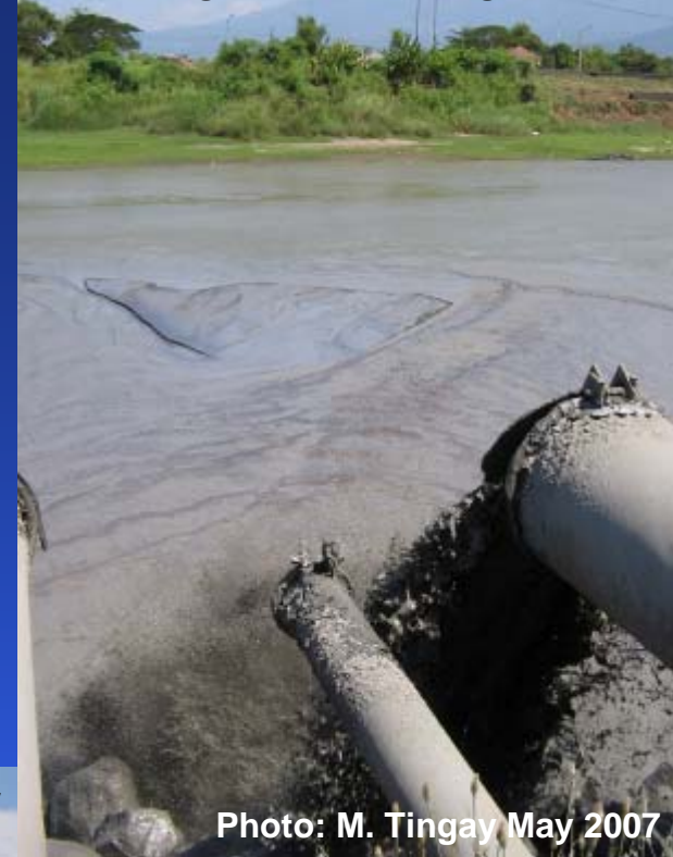
Sluicing into Porong River
